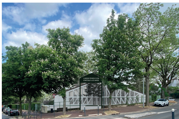
© Cabinet AJILE architectes / Archi : David LOVERA
